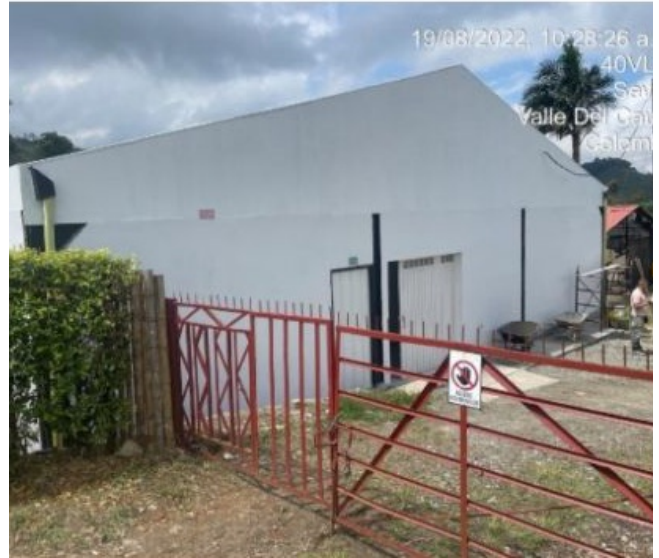
Production facility, Hacienda Flandes, Colombia.
