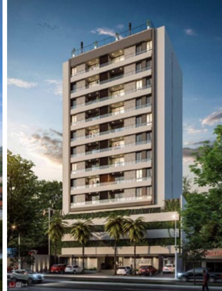
INFINITY BUILDING Structural detailed design (co-execution with Eng. Jesús Jiménez) Area: 5,800 m 2 Asunción · Paraguay
