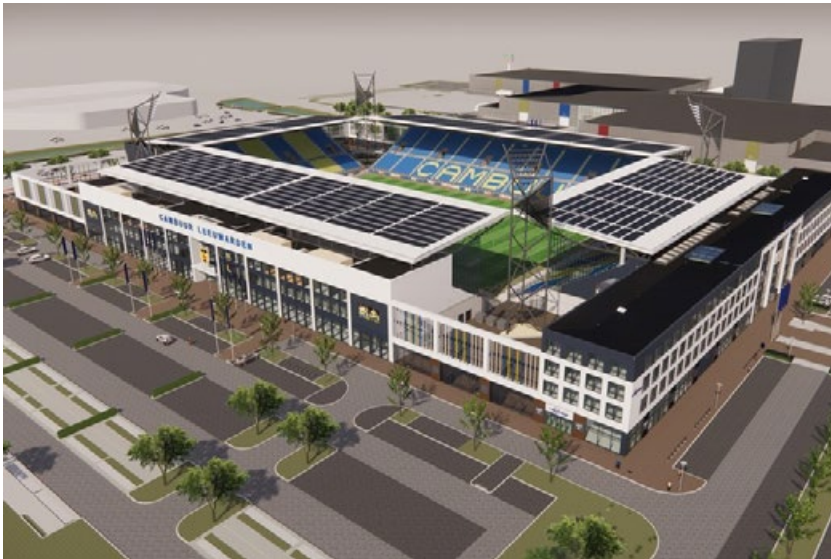
CAMBUUR Detailed design of a precast concrete and steel structure. Area: 23,000 m 2 Leeuwarden - The Netherlands
