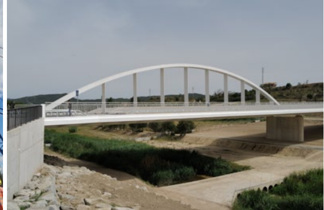
IGUALADA VIADUCT Catalonia - Spain
