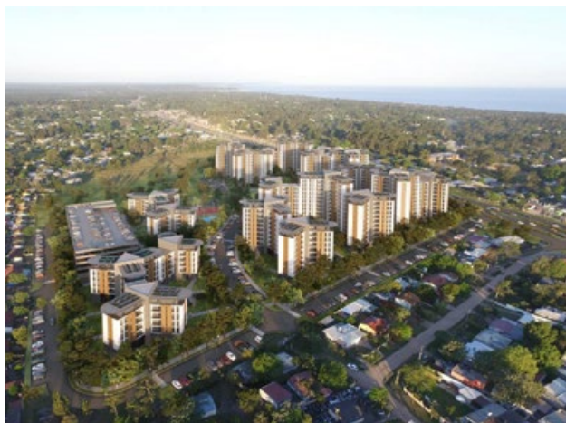
GIANNATTASIO HOUSING COMPLEX Preliminary structural design for modular precast Area: 95,000 m 2 Canelones · Uruguay
