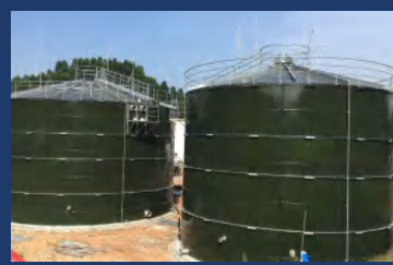
Conical Steel Roof
