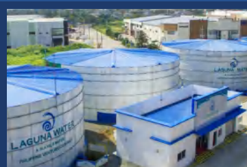
Aluminum Trough Deck Roof
