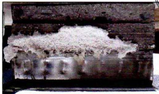
FIGURA 6: FOTOGRAFIA DE LA VIGUETA Y EMPASTE CON MALLA RF
