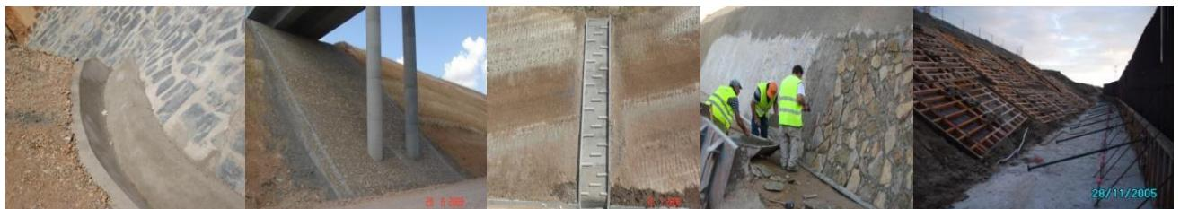
Platform: Drainage (excavations and landfills, pipes, hydrants, ditches, gutters boxes and bowls)
