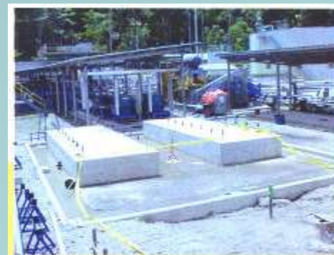
PETROBRAS-Constr. Base Bombas
