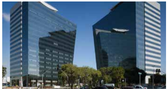
Rochaverá Corporate Towers (São Paulo - SP) Pre-construction, technology and erection of Tower C concrete structure, 25,000 m 3 , 3 underground floors and 34 storeys (17 months)
