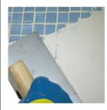
**Emplascem** is a two-component product in powder and liquid shape which are made each other achieving a plaster with thixotropic consistency.
