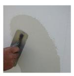
**Emplais** is a powder product based in cement to be mixed with water so as to form a plastic paste used for plastering, whitewash cracks and chippings on walls and ceilings, for interior use.
