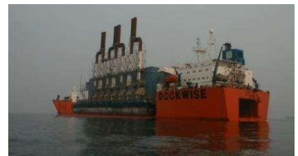
124 MW Power Barge, Guatemala
