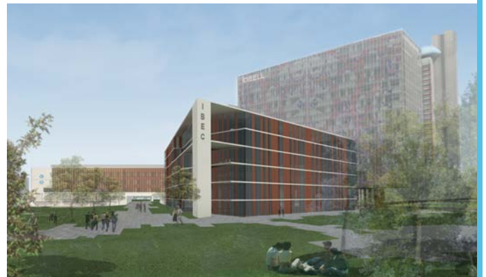
IBCB BUILDING. REFORMATION AND EXTENSION OF UNIVERSITY HOSPITAL OF BELLVITGE, BARCELONA, SPAIN 7.960 m 2 - IN PROGRESS
