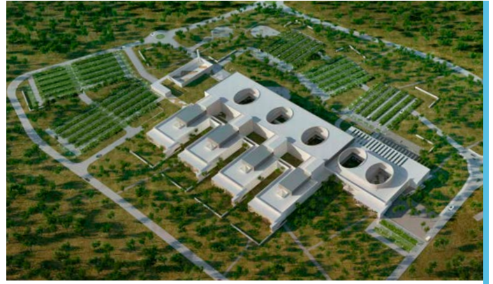
MONOPOLI - FASANO HOSPITAL BARI, ITALY 250.388 m 2 - IN PROGRESS
