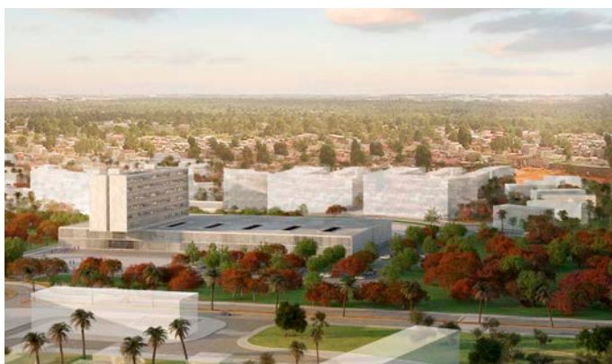
UNIVERSITY HOSPITAL IN LUANDA LUANDA, ANGOLA 43.550 m 2 - IN PROGRESS
