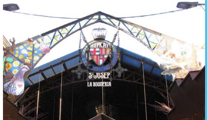
FIRST PHASE OF THE REFURBISHMENT OF THE "BOQUERIA" MARKET BARCELONA, SPAIN 816 m 2 - 6 MONTHS
