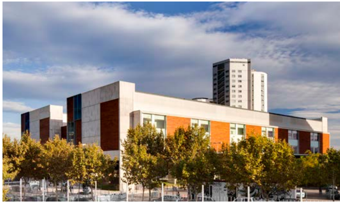
PRÍNCEPS D'ESPANYA EMERGENCY BUILDING, SURGICAL UNIT AND ICU BARCELONA, SPAIN 42.709 m 2 - IN PROGRESS
