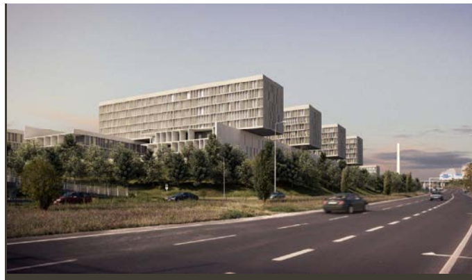
LISBOA ORIENTAL HOSPITAL LISBOA, PORTUGAL 240.000 m 2 - IN PROGRESS
