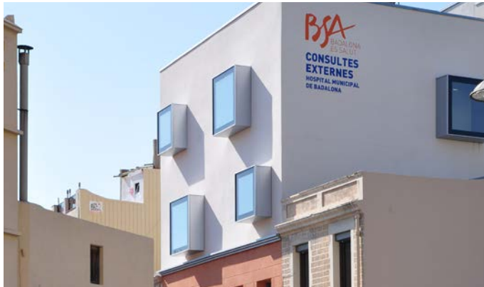
ESCALADA OUTPATIENT BUILDING, HOSPITAL OF BARCELONA BADALONA, SPAIN 1.126 m 2 - 14 MONTHS
