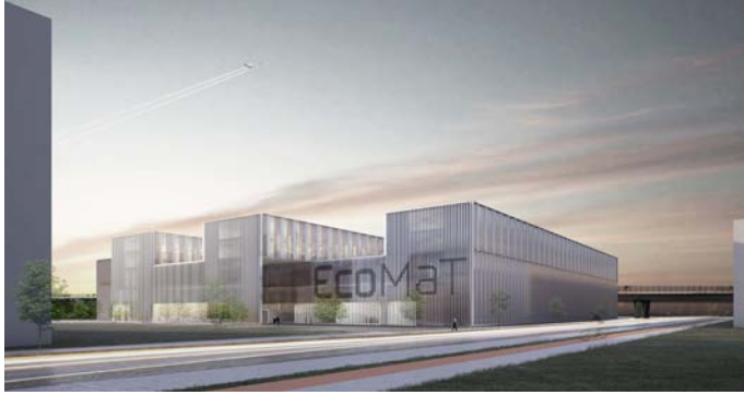
ECOMAT LABORATORY BREMEN, GERMANY 22.779 m 2 - IN PROGRESS
