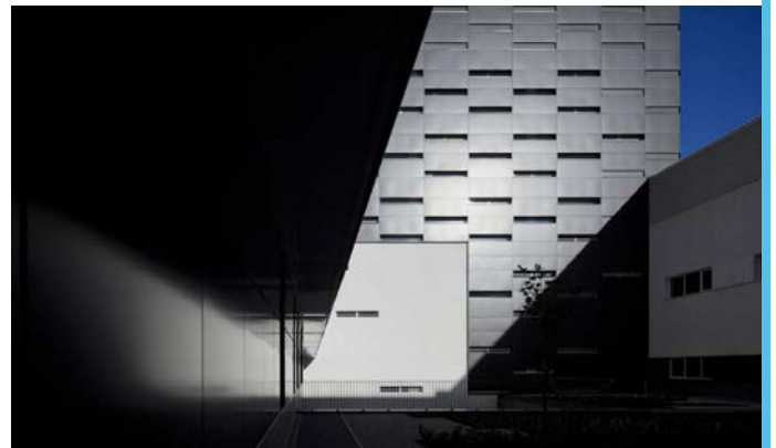
BEATRIZ ÂNGELO HOSPITAL LOURES, PORTUGAL 90.375 m 2 - 28 MONTHS
