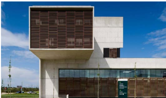
HOSPITAL IN DÈNIA DÈNIA, SPAIN 57.194m 2 - 25 MONTHS
