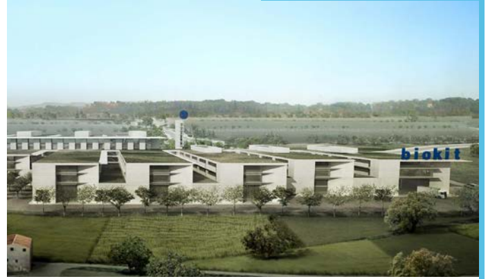
BIOKIT LABORATORY LLIÇA DE MUNT, SPAIN 60.000 m 2 - IN PROGRESS
