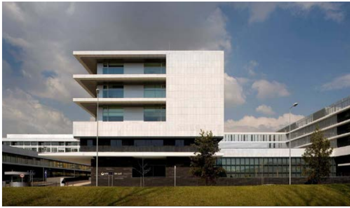
HOSPITAL DA LUZ LISBOA, PORTUGAL 50.230m 2 - 24 MONTHS
