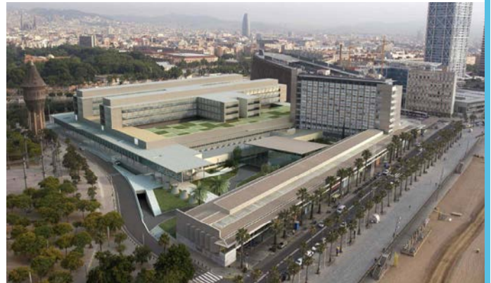
EXTENSION OF HOSPITAL DEL MAR BARCELONA, SPAIN 103.527 m 2 - IN PROGRESS
