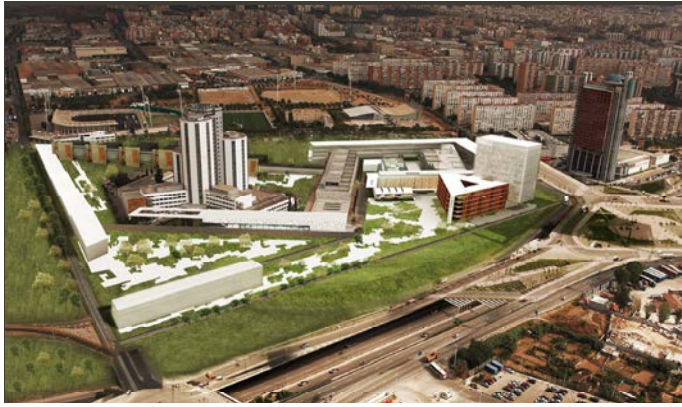
HOSPITAL AND UNIVERSITY IN BELLVITGE BARCELONA, SPAIN 88.850 m 2 - IN PROGRESS
