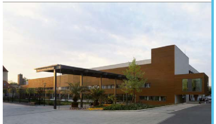
HEDWIGSHÖHE HOSPITAL BERLIN, GERMANY 30.000 m 2 - 48 MONTHS
