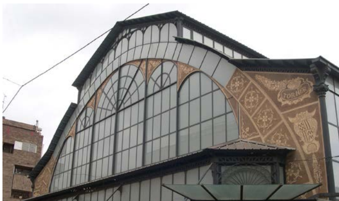
IMPROVEMENT AND PROVISIONAL FACILITY OF TORNER MARKET BADALONA, SPAIN 11.491 m 2 - IN PROGRESS
