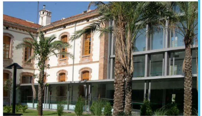
CASTELLÓ REGIONAL HOSPITAL CASTELLÓ DE LA PLANA, SPAIN 37.809 m 2 - 40 MONTHS
