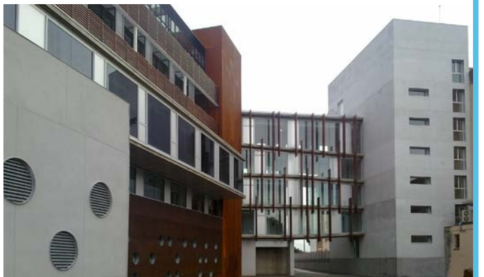
SANT BERNABÉ HOSPITAL BERGA, SPAIN 5.923 m 2 - 20 MONTHS
