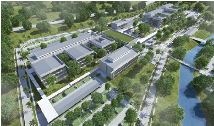
CAMPUS ANTENAS PANAMA, PANAMA 28.710 m 2 - IN PROGRESS
