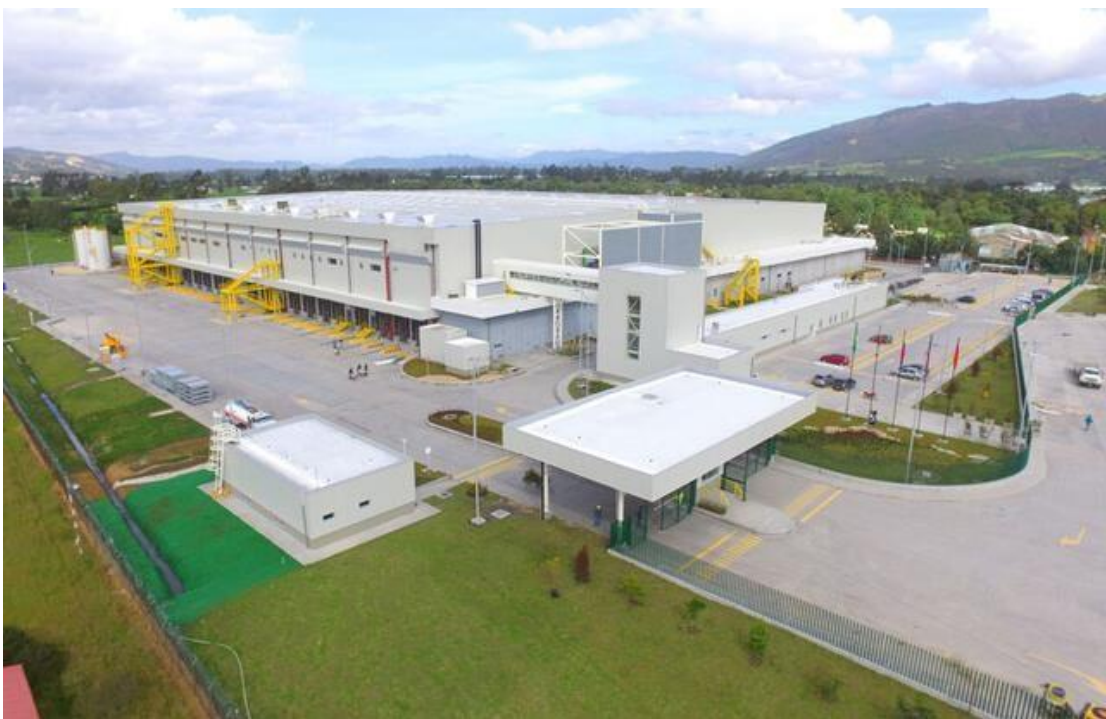
WAREHOUSE ARA - GACHANCIPA
