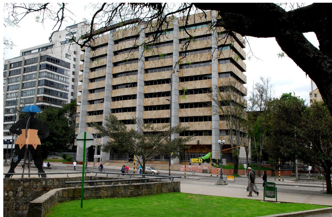
ECOPETROL OFFICE REINFORCEMENT - BOGOTÁ
