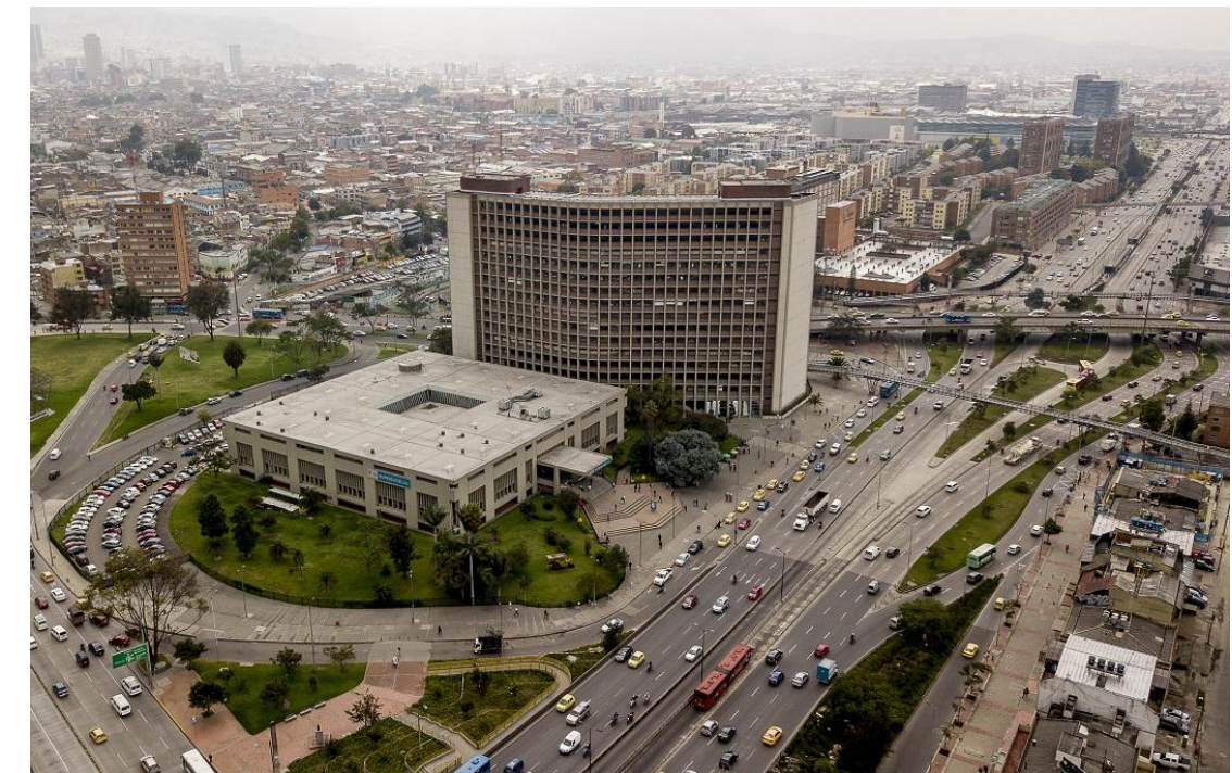
REINFORCEMENT SUPERCADDE - BOGOTÁ
