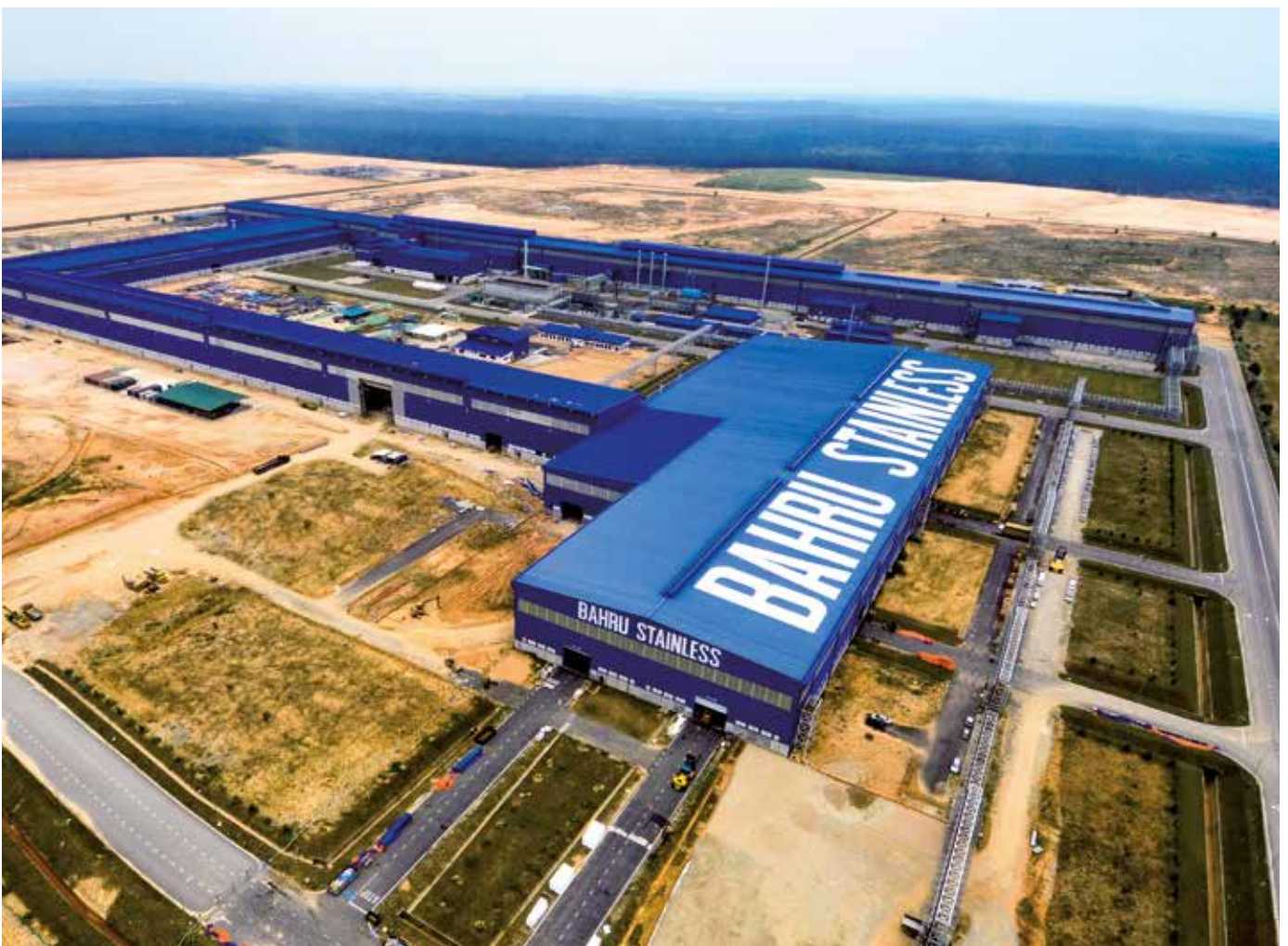
Stainless steel manufacturing plant in Malaysia. Acerinox
