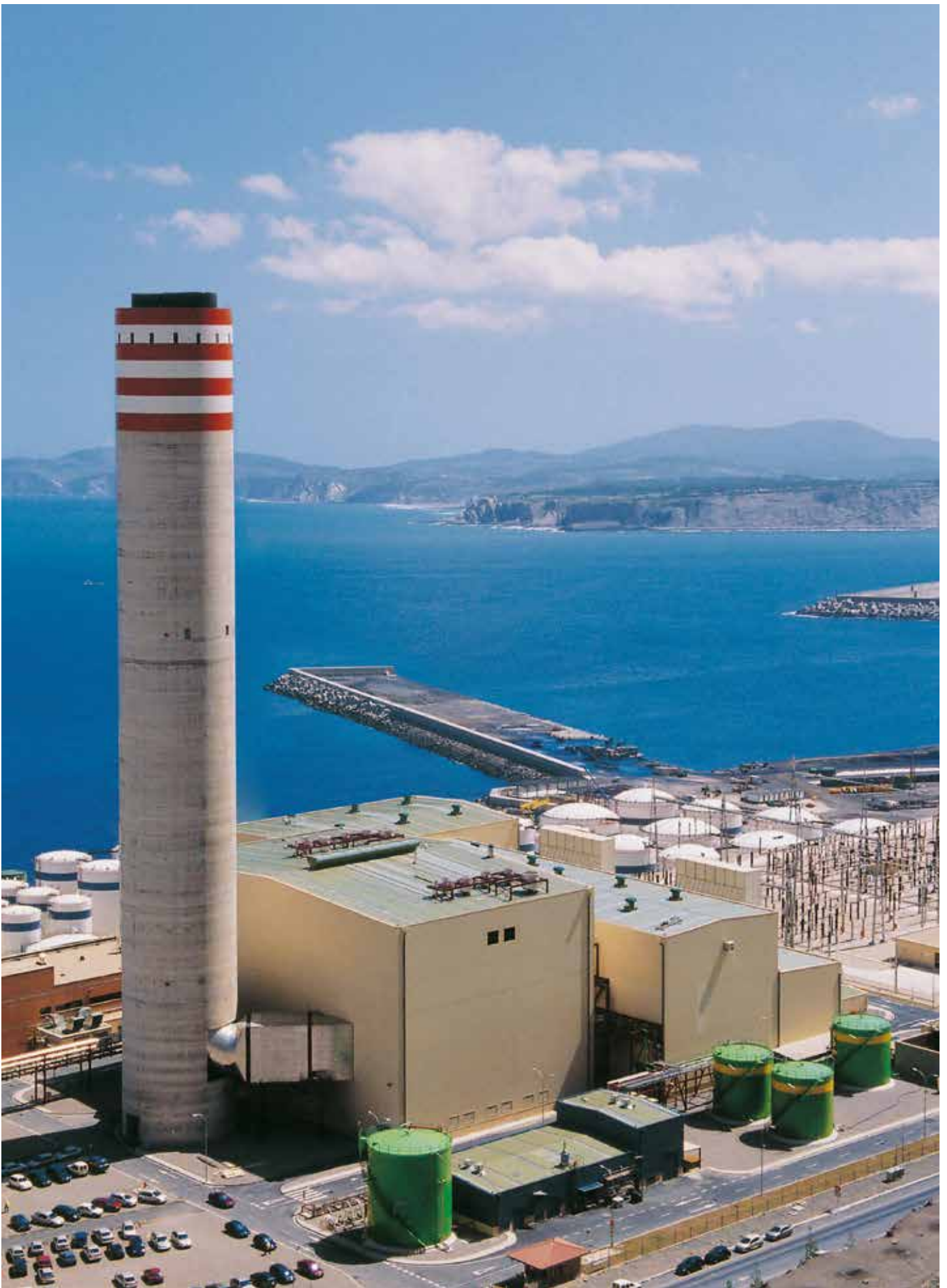
Bizkaia Bay combined cycle Power Plant
