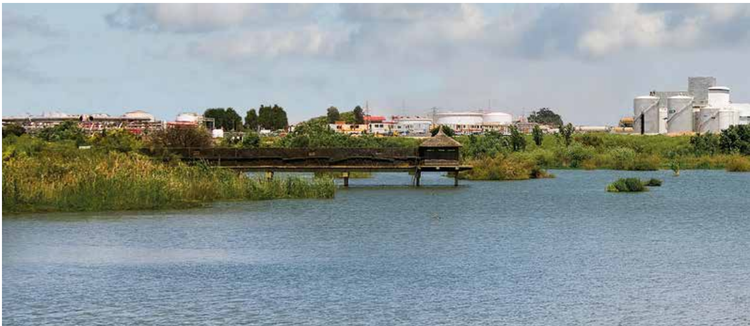
Biodiesel plant in Huelva
