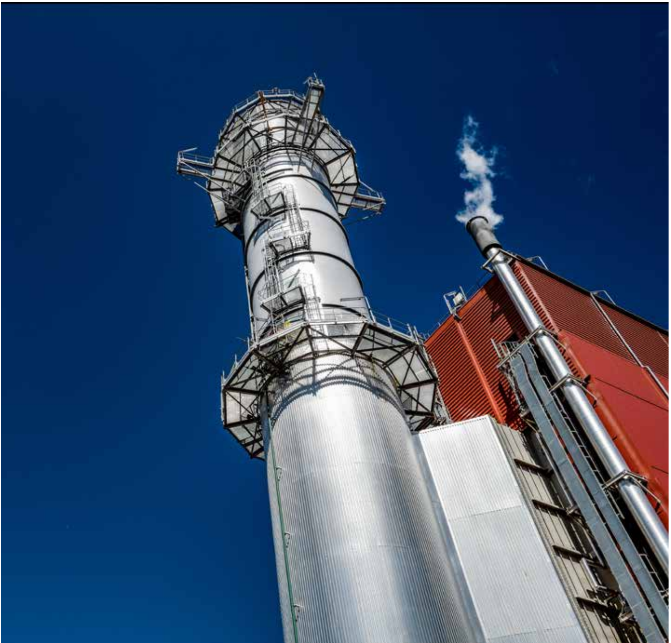
Combined cycle power plant of Bouchain, France
