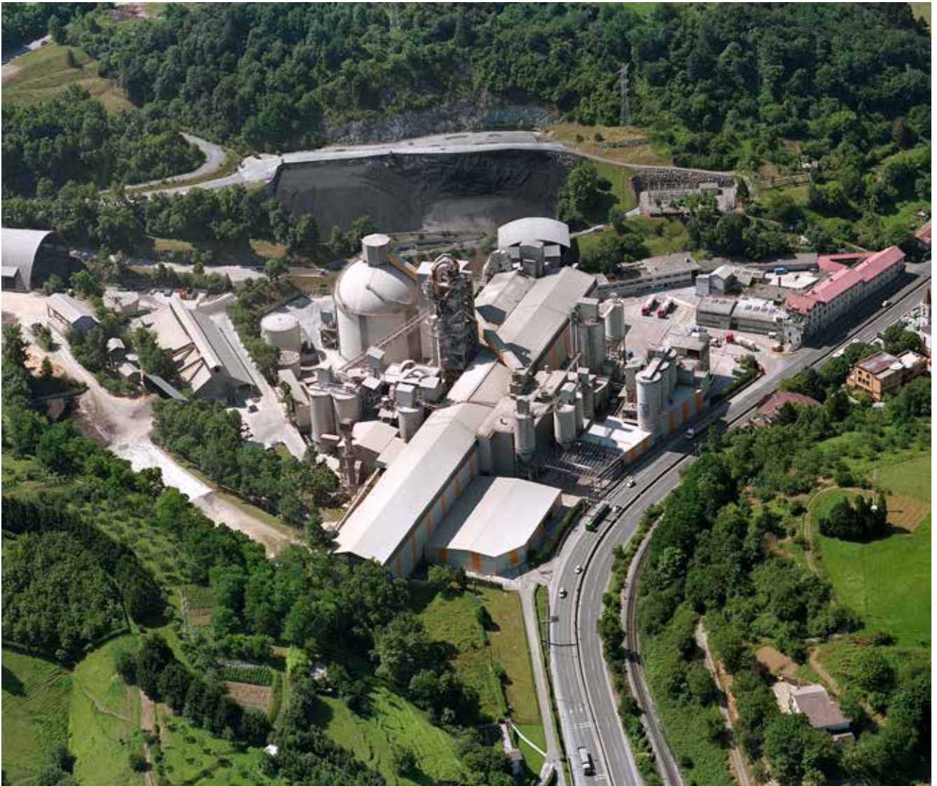
Cement plant in Gipuzkoa
