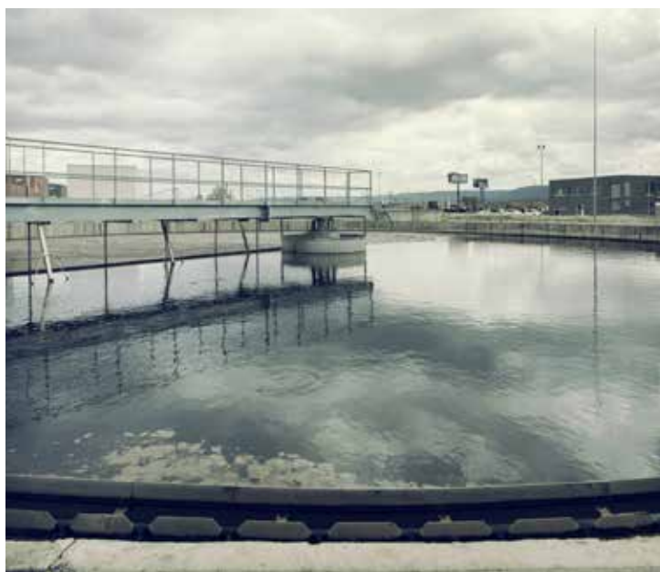
Sanitation of Zonguldak Municipality - Turkey
