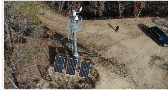
'23.10. Drone Video Transmission of Trailer TVWS Base Station
