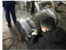
Weld Seam UT/MT
